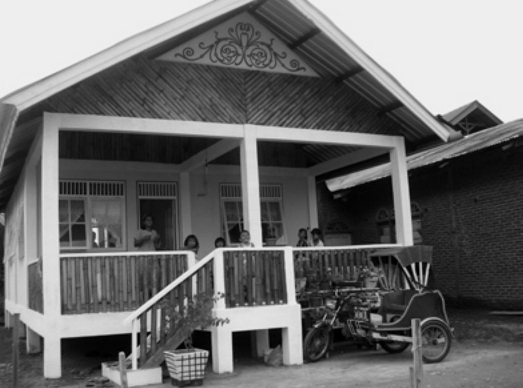
Fondation de France raised more than €20 million following the 2004 tsunami in Asia. This is one of the houses built as a result. Architectes de l'Urgence
